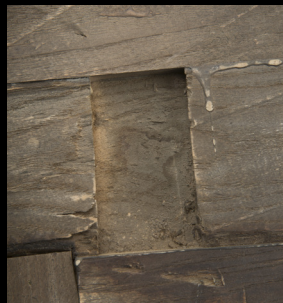
Hinge marks (underside)
